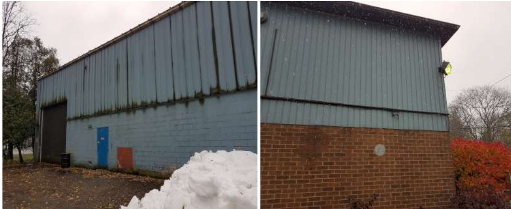
(a) Exterior block wall (b) Exterior wall with brick veneer
