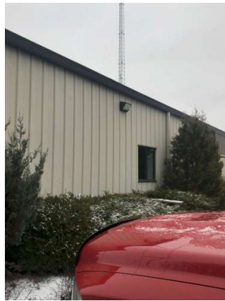
(a) Exterior wall
