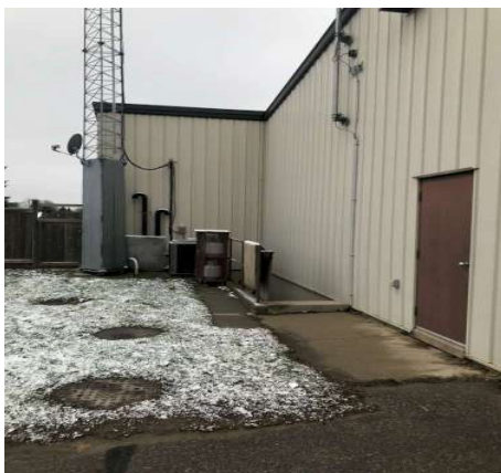
(a) Exterior door
