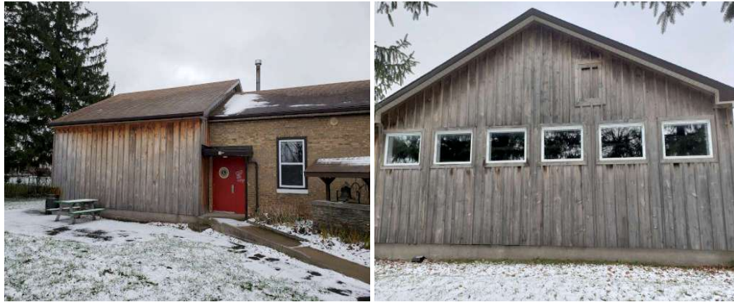
(a) Exterior brick and wood wall
