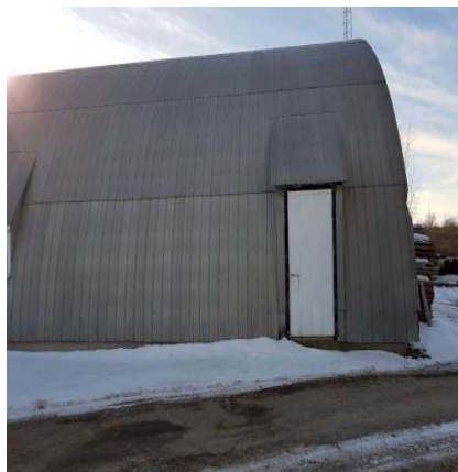
(b) Quonset hut exterior wall
