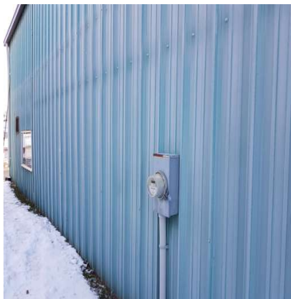
(a) Main building exterior wall
