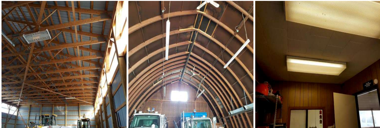
(a) Garage fluorescent fixtures
