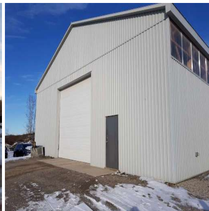
(c) Storage building exterior wall
