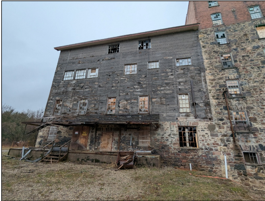
Photograph 3: Nail-Lam Portion from Exterior
