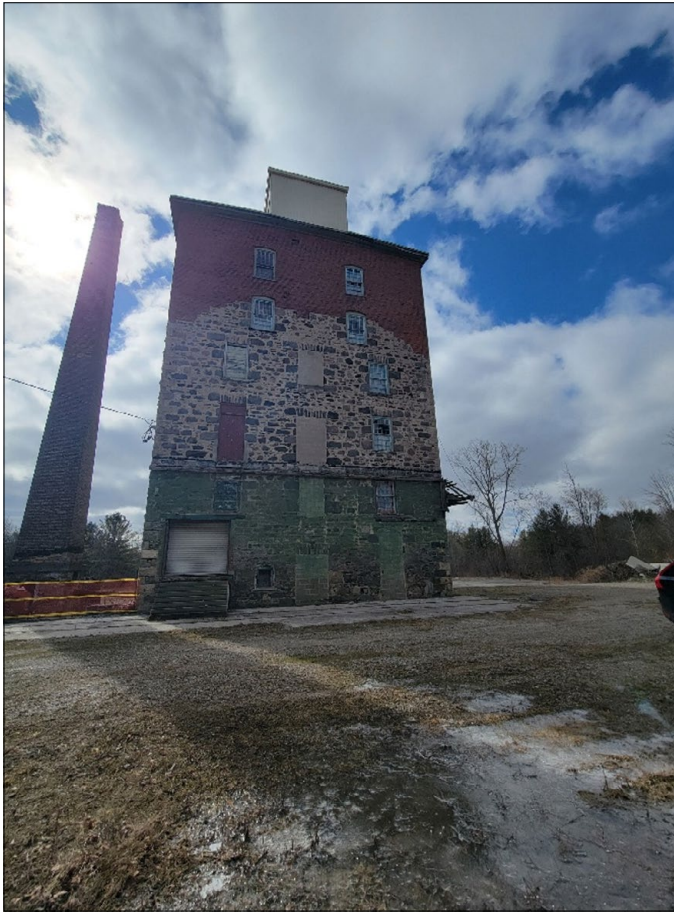
Views of the north elevation of the building showing the four storey historic stone mill (1850) and upper brick addition (1890s). (TBG, 2026).
