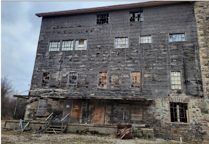
Figure 21. East Elevation (Plank/Nail-lam Section)
