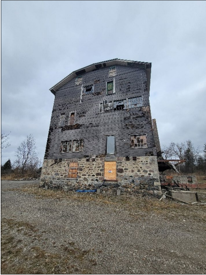
Views of the south elevation which includes the plank/ nail-lam timber structure which constitutes the rear wing.
