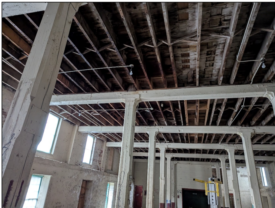
Photograph 1: Interior Wood Framing
