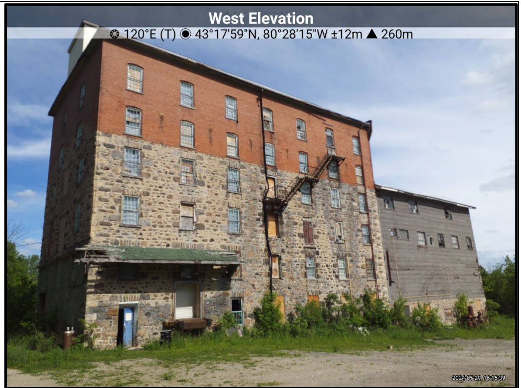
Photo 1: May 29, 2024 The west side of the old mill structure.
