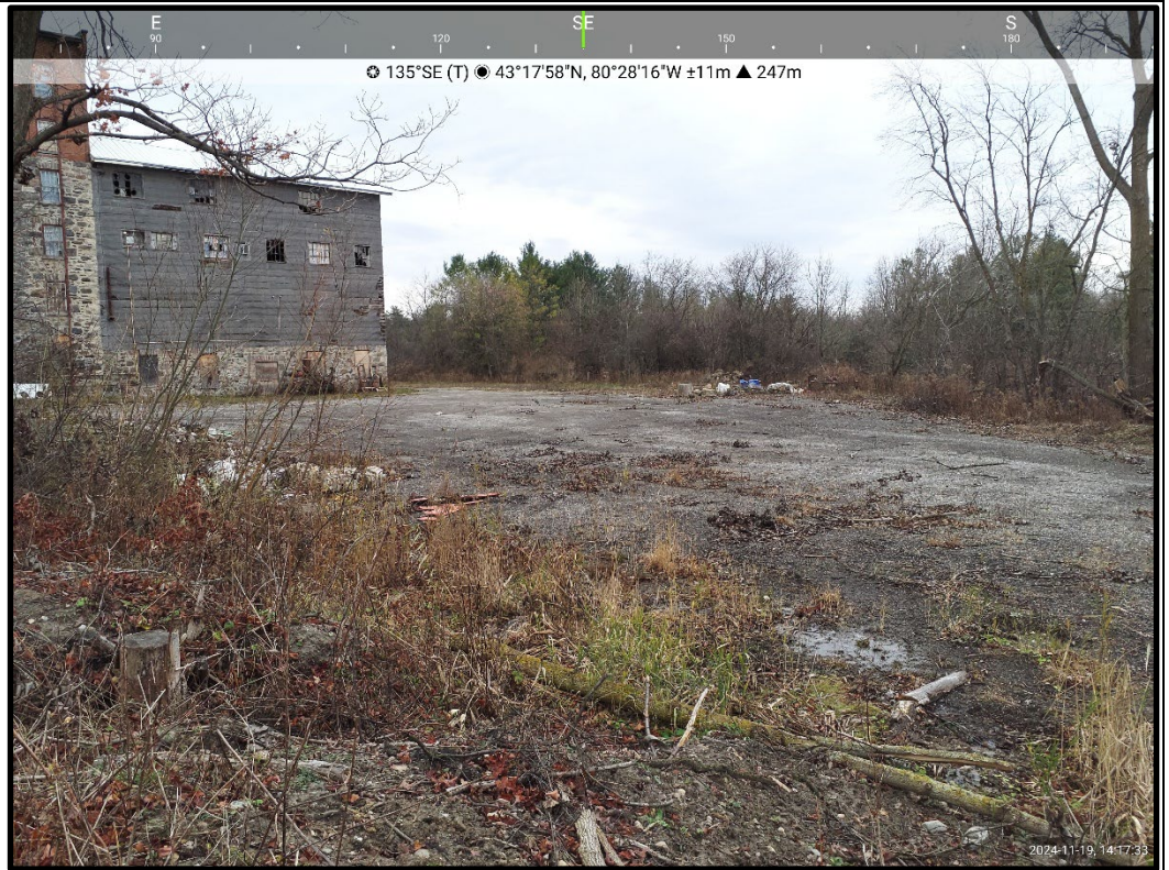
Photo 9: Nov 19, 2024 Southwest portion of the Site, showing existing gravel parking/loading area, looking southeast.
