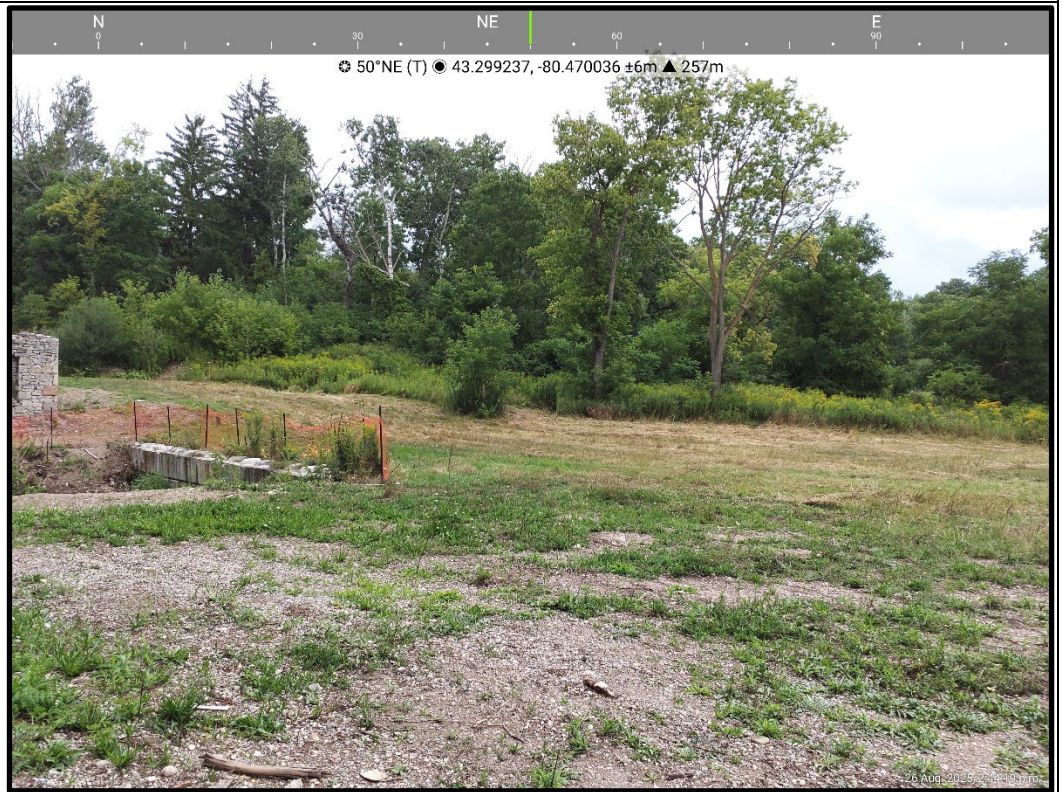
Photo 16: Aug 26, 2025. The former spillway east of the mill and treed right of way to the east of the Site, looking northeast.
