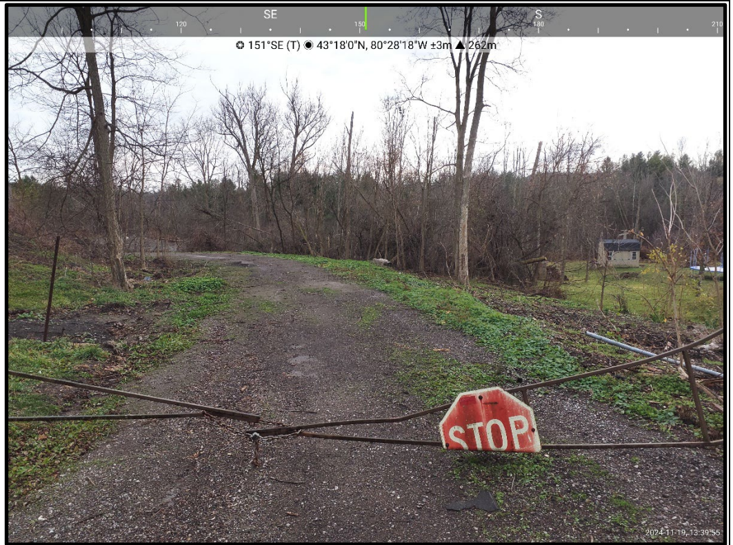
Photo 3: Nov 19, 2024 Existing laneway, view from road looking south, showing some of the tornado damage to the trees.
