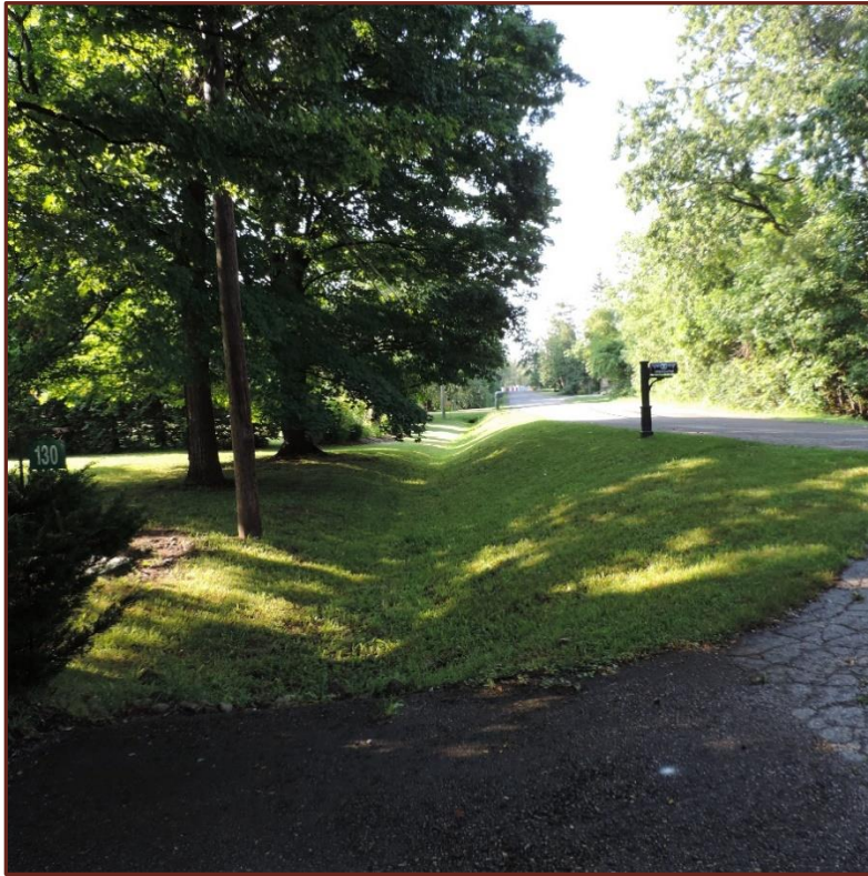
Photo 13. A view of the ditch and culverts under the neighbours' driveways.
