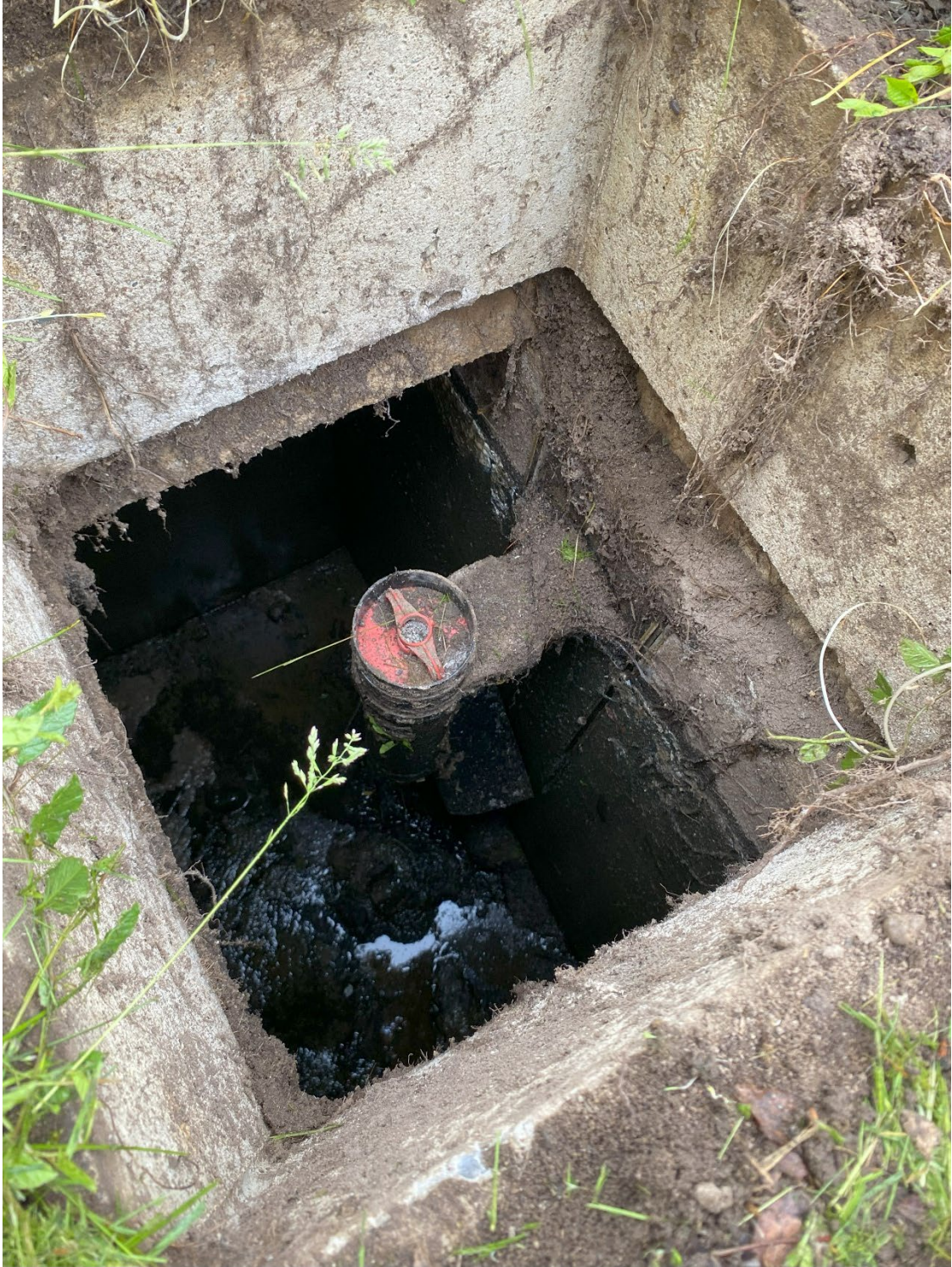
3 – Septic tank outlet side with effluent filter.
