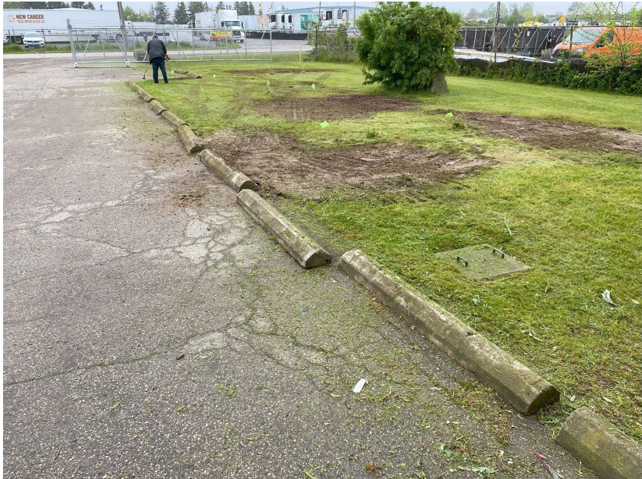
1 - Surface of leaching bed showing test pit excavation areas.
