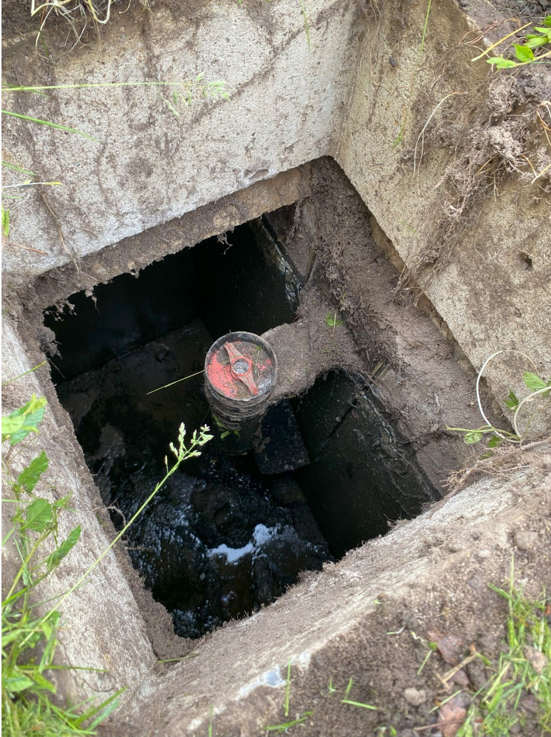
3 – Septic tank outlet side with effluent filter.
