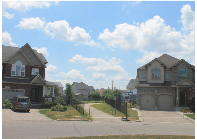
Examples of residential lots abutting walkways/trail systems.
