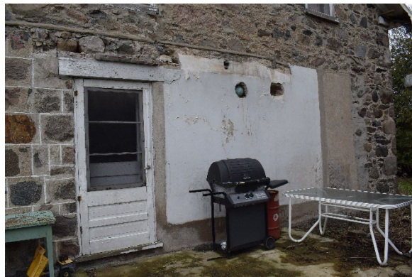
Plate 22: Concrete replacement wall, looking south
