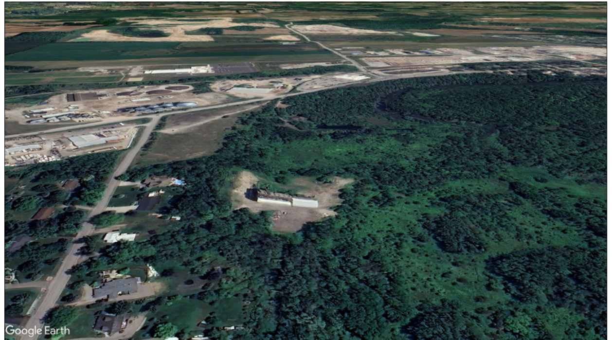
Figure 5. Surrounding Context: Aerial View East (Google Earth)
